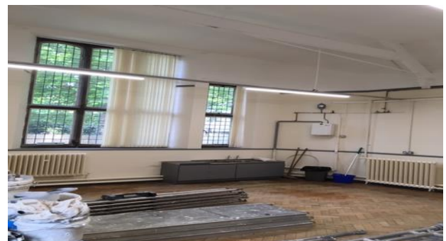
Room 17 gets a fresh new look too
